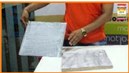
Step 9 : BERGA PVC GLUE to be applied to both the SURFACE and stick together immediately.
