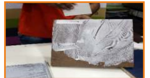
Step 8 : Apply THIN layer of the glue on the surface of the plywood which has been scratch.
