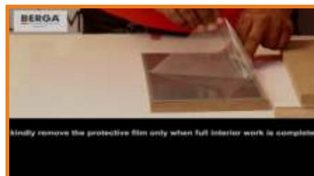
Step 15 : Kindly remove the protective film only when full interior work is completed.
